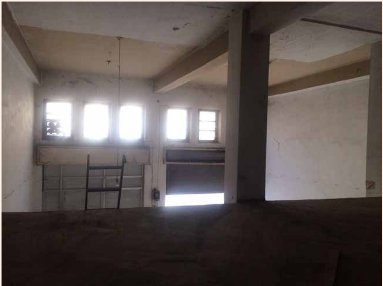
EVENT VENUE - TURBO DESIGN STUDIO - UNDER CONSTRUCTION
